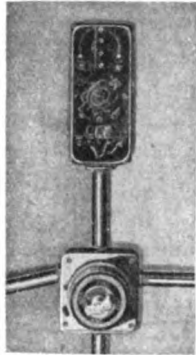
SHOWING THERMOSTAT AND SWITCH CONTROL
